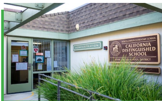
Bonita Canyon Elementary School, Irvine CA
