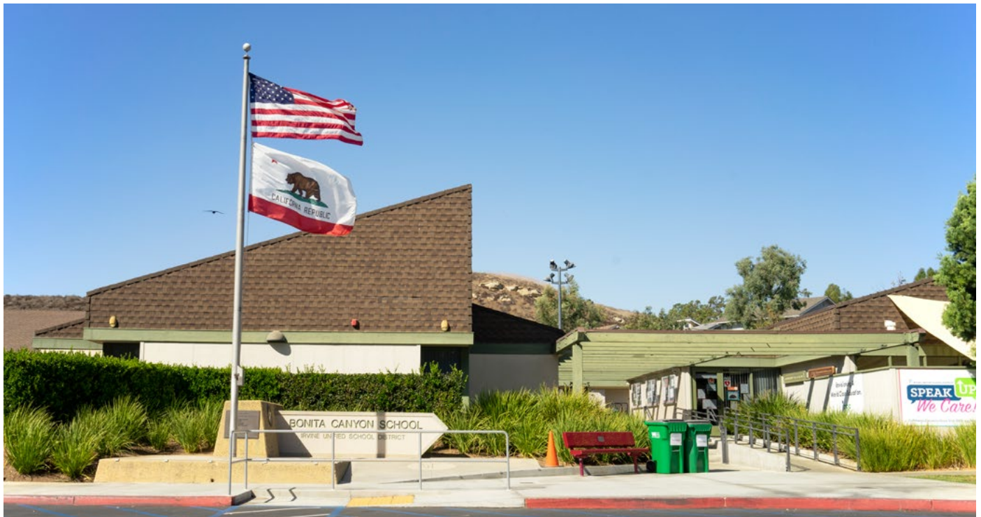
Bonita Canyon Elementary School, Irvine CA
